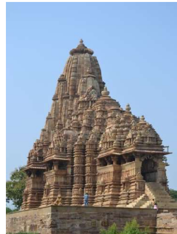
Figure 13: Images showing the exterior of the Kandariya Mahadev temple highlighting the effect of the jagged external geometry created by plan form (by authors).
