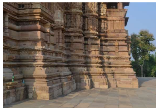
Figure 16: Image showing base of Kandariya Mahadev temple where the emanating plan form is visible (by authors).
